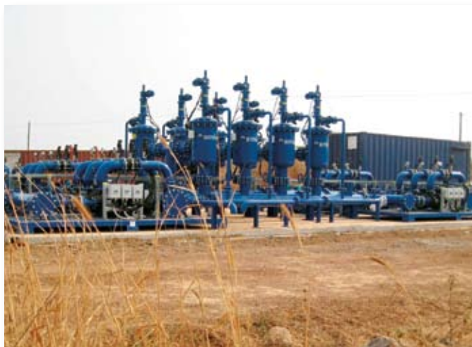
Angola, Waku Kungo, Complete water supply (Drinking water, Industrial & irrigation)
