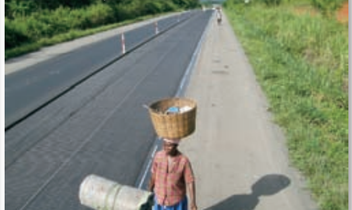
Reinforcement of asphalt structure - Ghana
