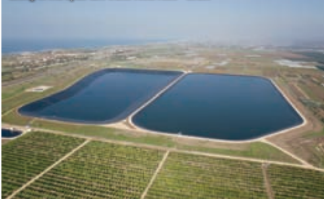
Lining of Ma'ayan Tzvi water reservoirs - Israel
