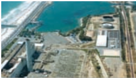
Carlsbad, USA - the largest desalination plant in the western hemisphere
