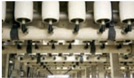
Sorek, Israel - Innovative vertical membrane arrangement
